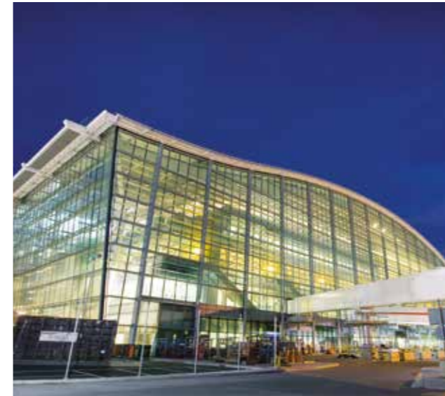
Heathrow Airport – Terminal 5 Location: London, U.K. Architect: Richard Rogers Contractor: Mansell
